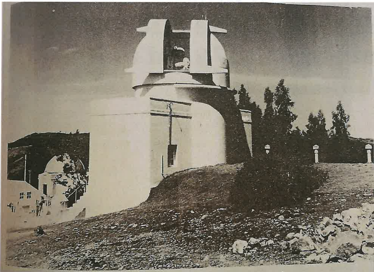
The Kodaikanal Solar Observatory back in the day. (Via 'Hundred Years of Weather Service', IMD)
